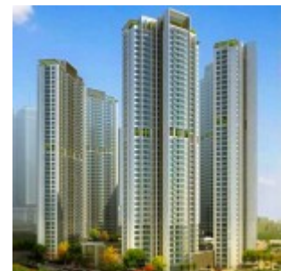
Tower TA Residences
