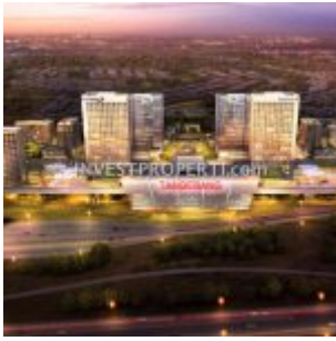
Lavon Swan City Cikupa Tangerang MRT Station
