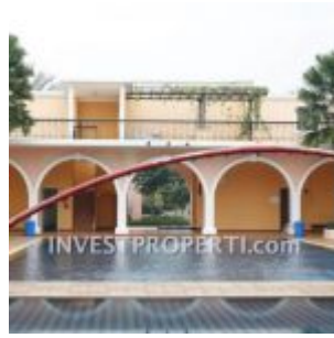
Club House Alicante Village
